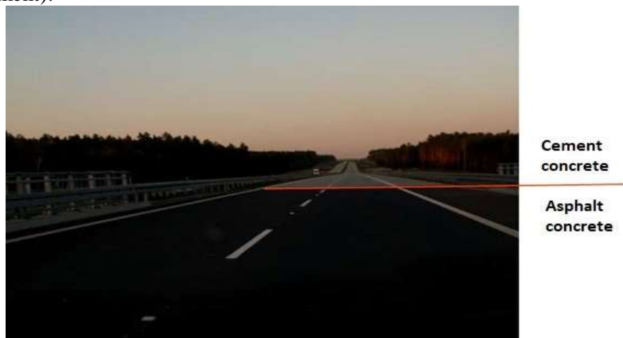
Fig. 1. Comparison of the brightness (visibility) of a cement concrete and asphalt concrete road.
