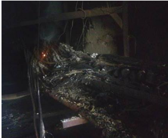
Fig. 11. Photographs of cables in the tunnel after finishing the experiment
