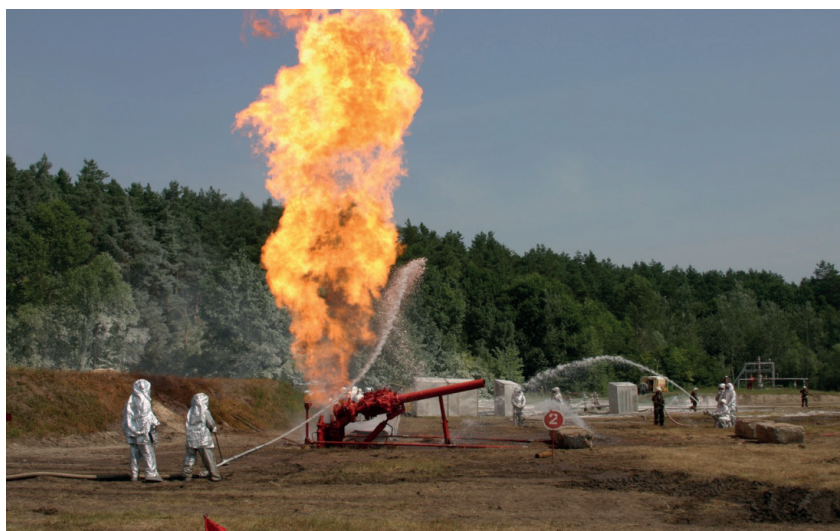
Fig. 9. Installing the BOP Source: Own elaboration.
